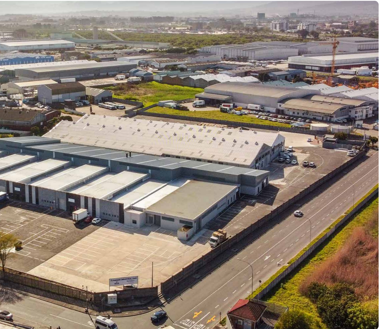
Vega Properties: Newly developed Radnor Industrial Park.
